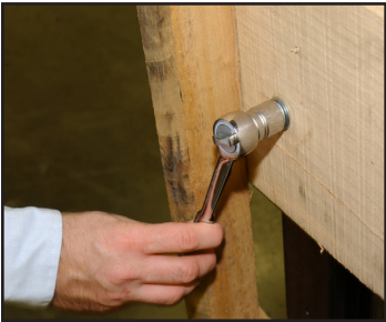
Removing skid from bottom of cabinet.
